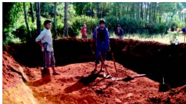
Fig 11 Excavation of Jalkund in progress
