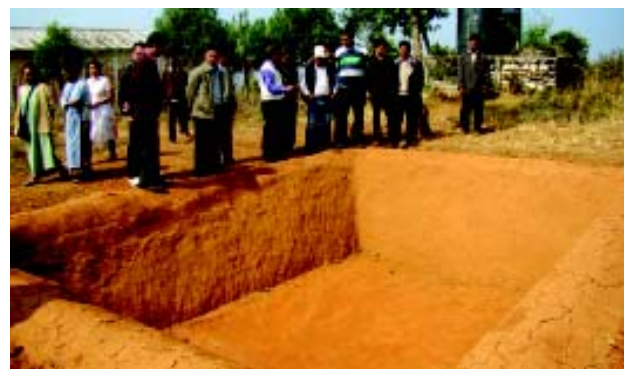
Fig 12 Monitoring the Jalkund after the excavation
